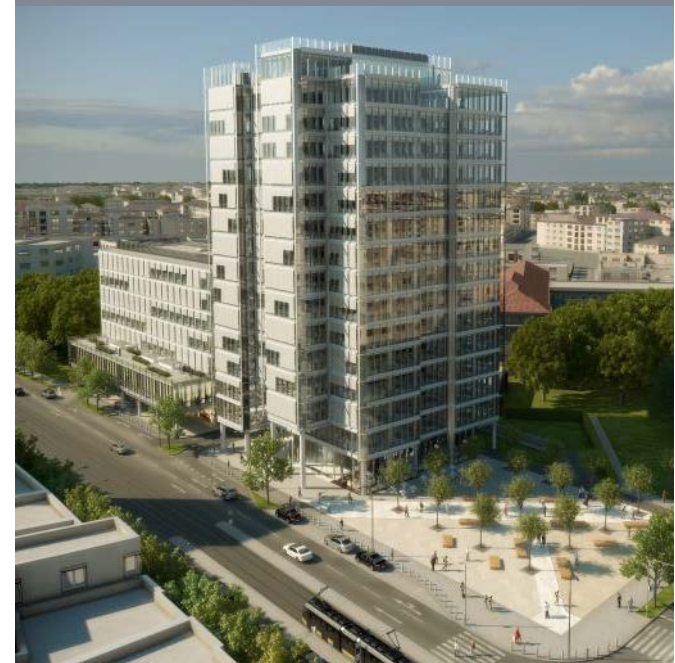
Under construction: The Mark
